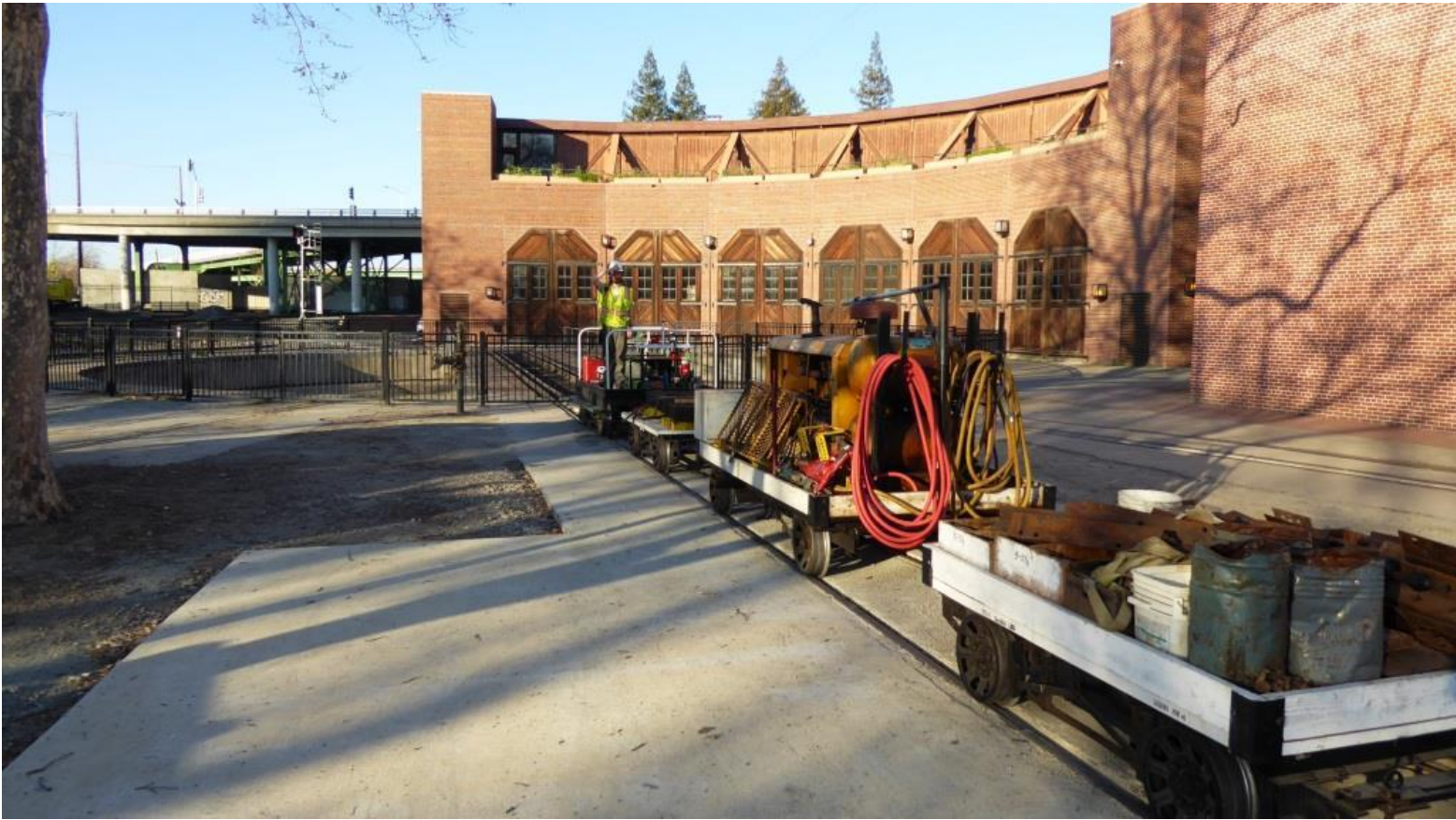
Matt on the A-6 motorcar, who has just pulled the entire work-train consist out of the container, stands at attention awaiting orders
