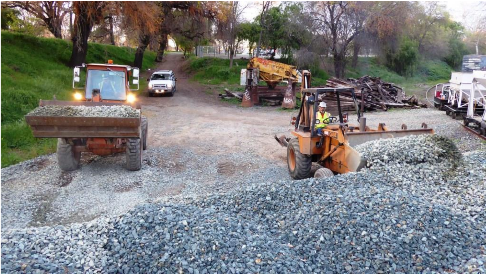
Frank in the front-end loader and Ed on the back-hoe scoop-up rock for loading into the hopper-cars
