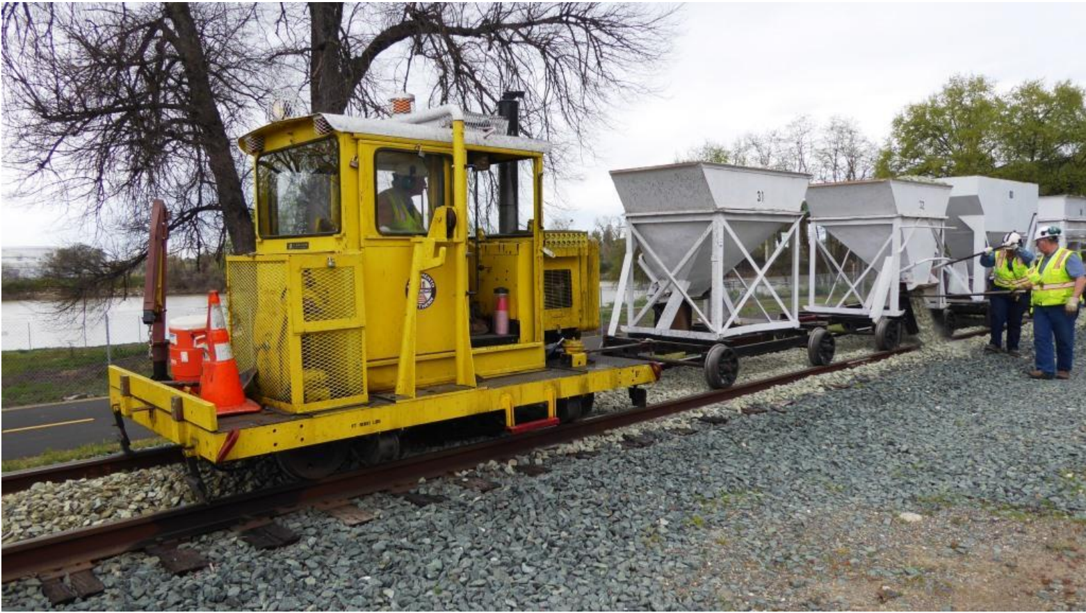
The ballasting operation in progress
