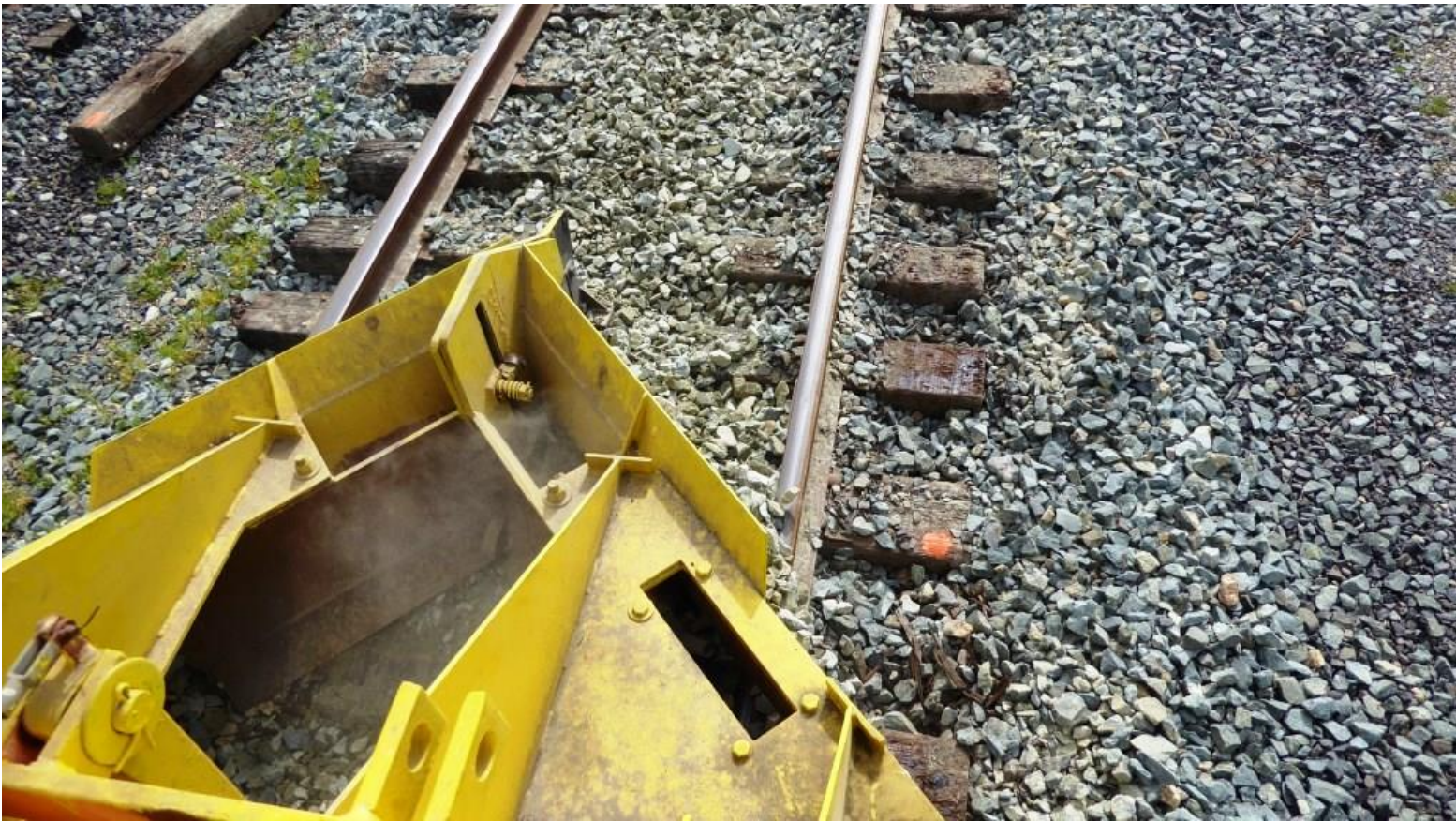
The plow of the ballast regulator as it plows rock over the rails
