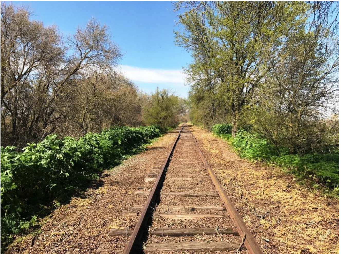
Looking north on the Hood Line at MP 11.6 after the Weedies finished mowing
