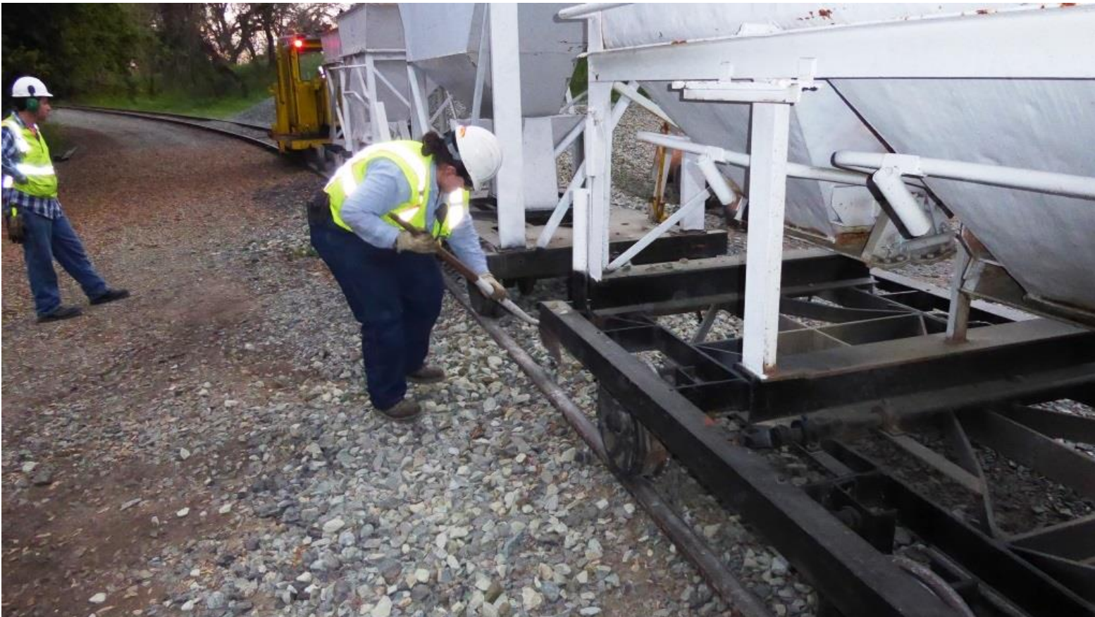
Despite being her birthday, Heather keeps on working and clears rock from the head of the rail with the broken-handled shovel
