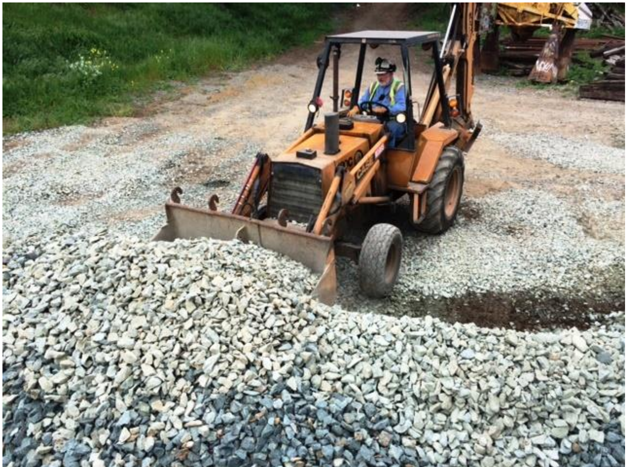
Meanwhile, Frank on the back-hoe at Setzer, loads another round of rock into the hoppers
