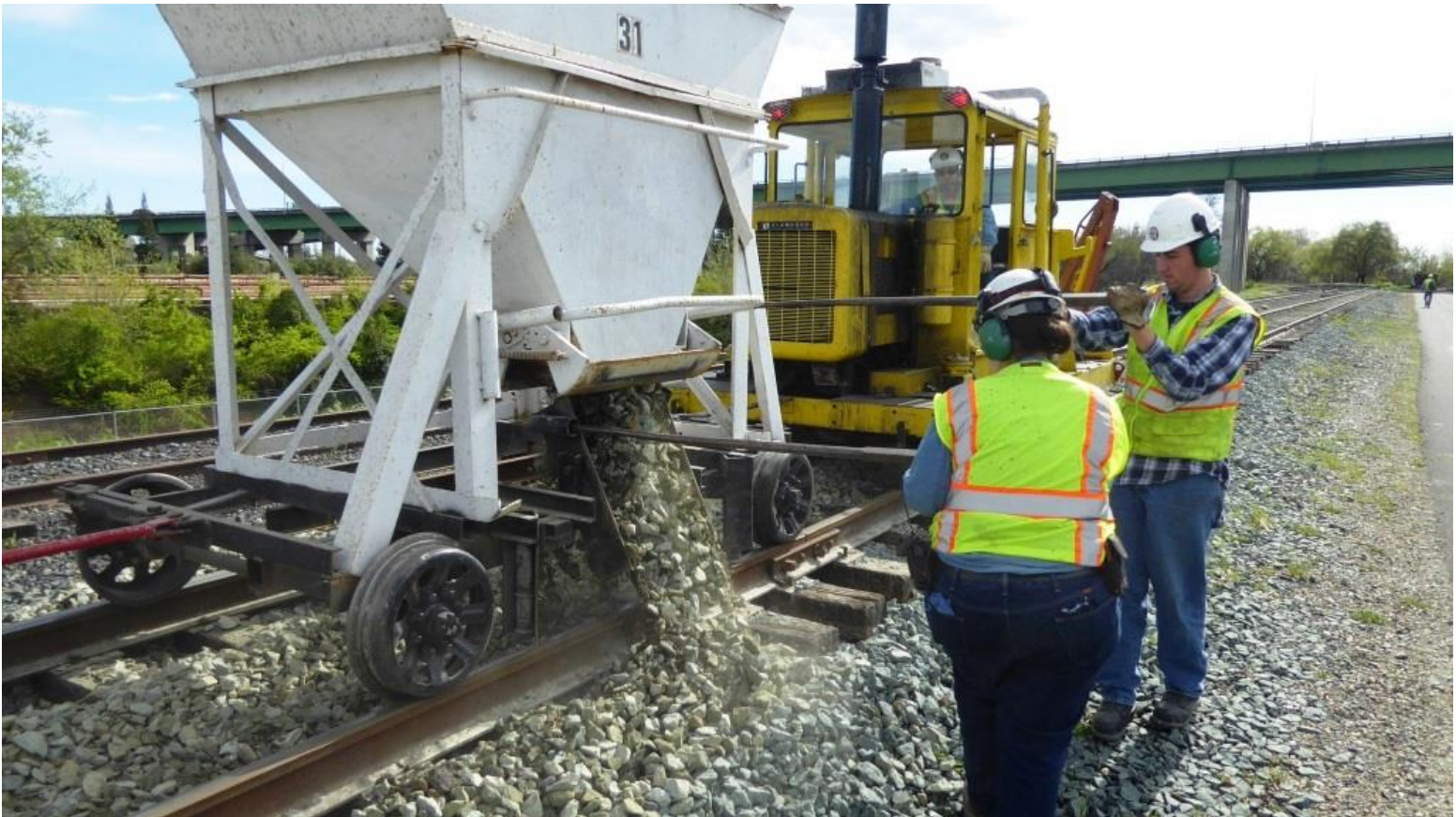
Heather and Weston discharge another hopper of rock
