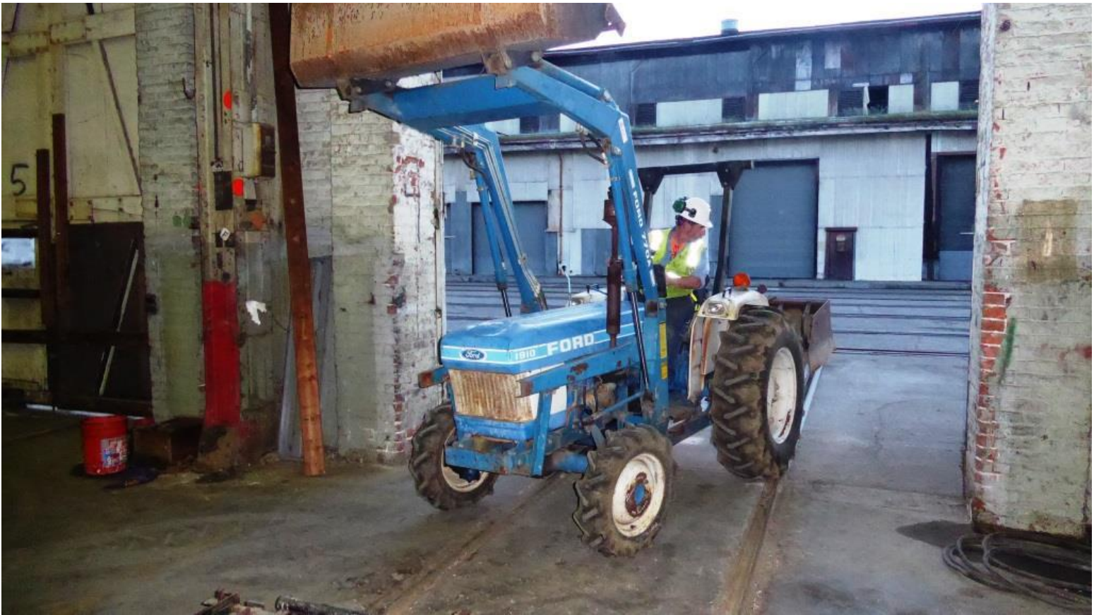
Now that it's been repaired Joe takes the MOW Team's blue tractor back to the Boiler Shop
