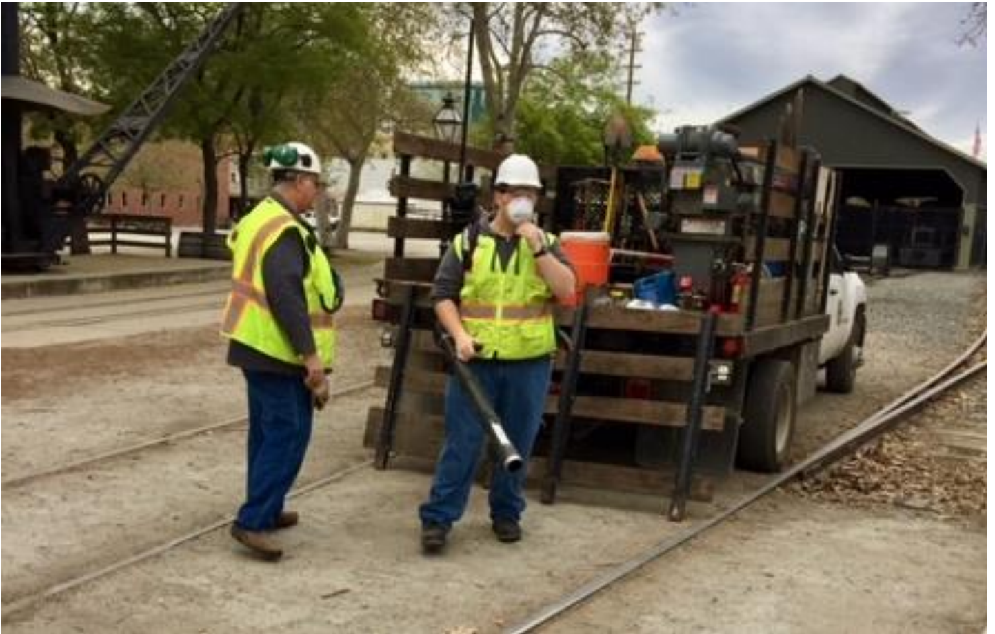
The lone picture from Saturday's switch repair: Josh dons the "huff-'n'-puff" machine to blow organic debris from around the switch
