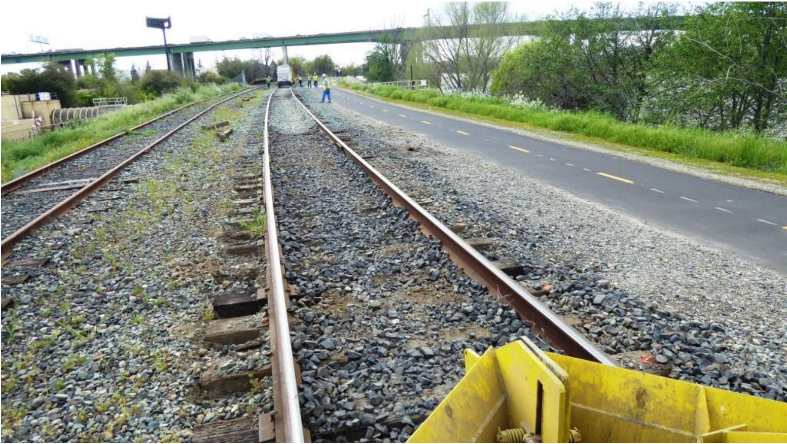
The ballast regulator awaits the arrival of the ballast-hoppers for round-two of rock-dropping
