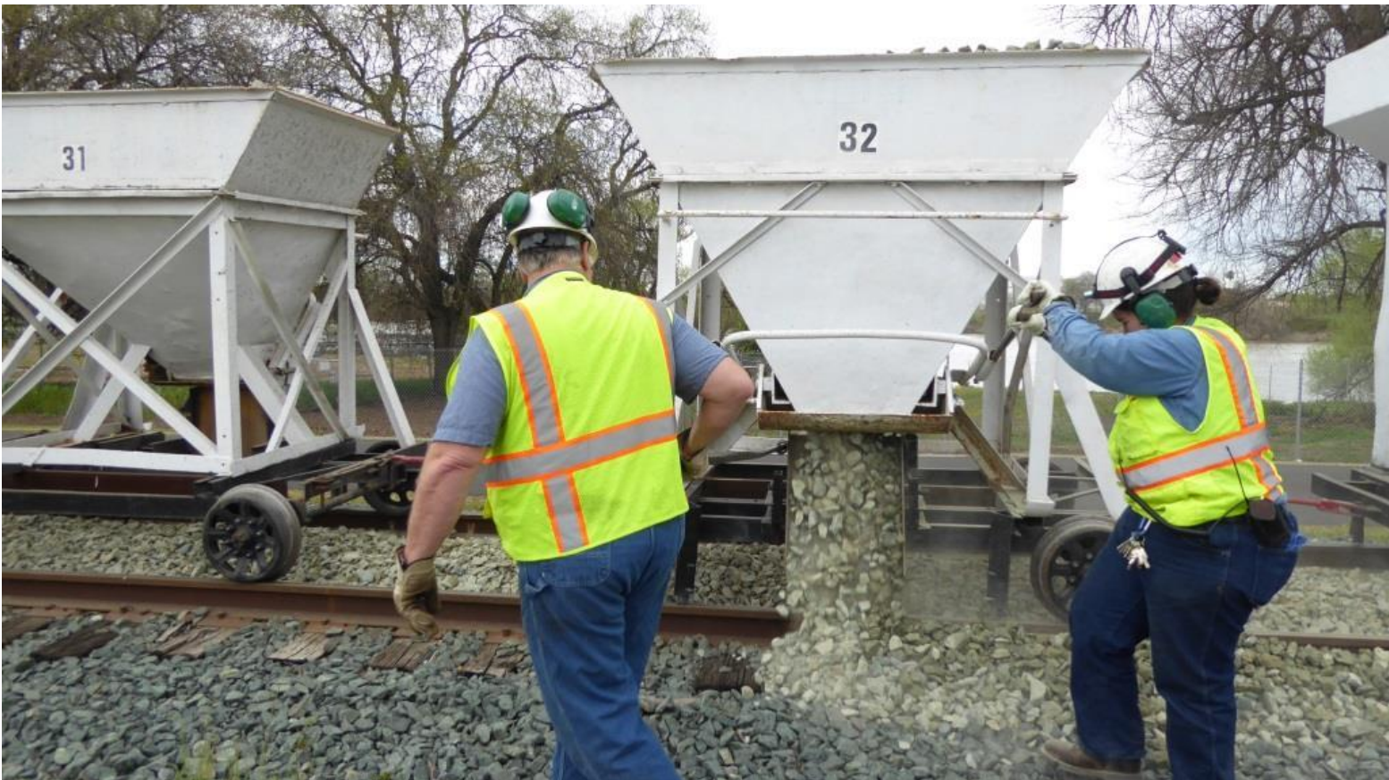
Chris and Heather drop rock along the east side of the track
